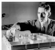
In 1951 Claude Shannon, founder of Information Theory (Collins, 2002), developed one of the first learning machines – a life-size mouse controlled by magnetic relay circuits adapted from telephone circuits. The mouse was able to learn to traverse a 25-square maze from any point in the maze. The maze could be modified, and the mouse would relearn the portions of the maze that had changed (Klein, 2018).
